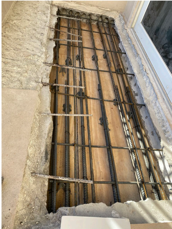
Picture 1: Unit 103 concrete repair
